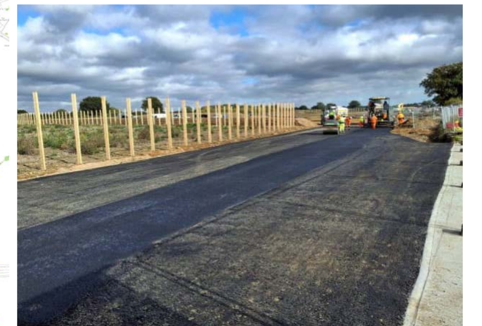
Construction of Phase 1 now underway below (see image below)
