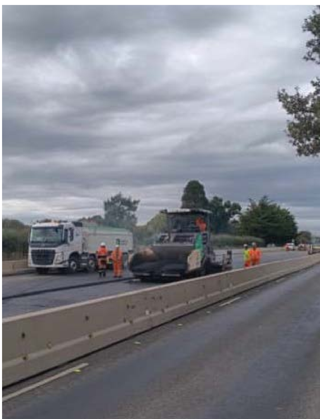
Above: A133 Lane realignment construction underway
